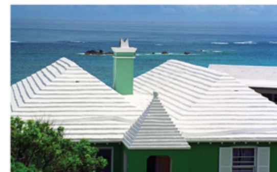
Limestone roofs of Bermuda
