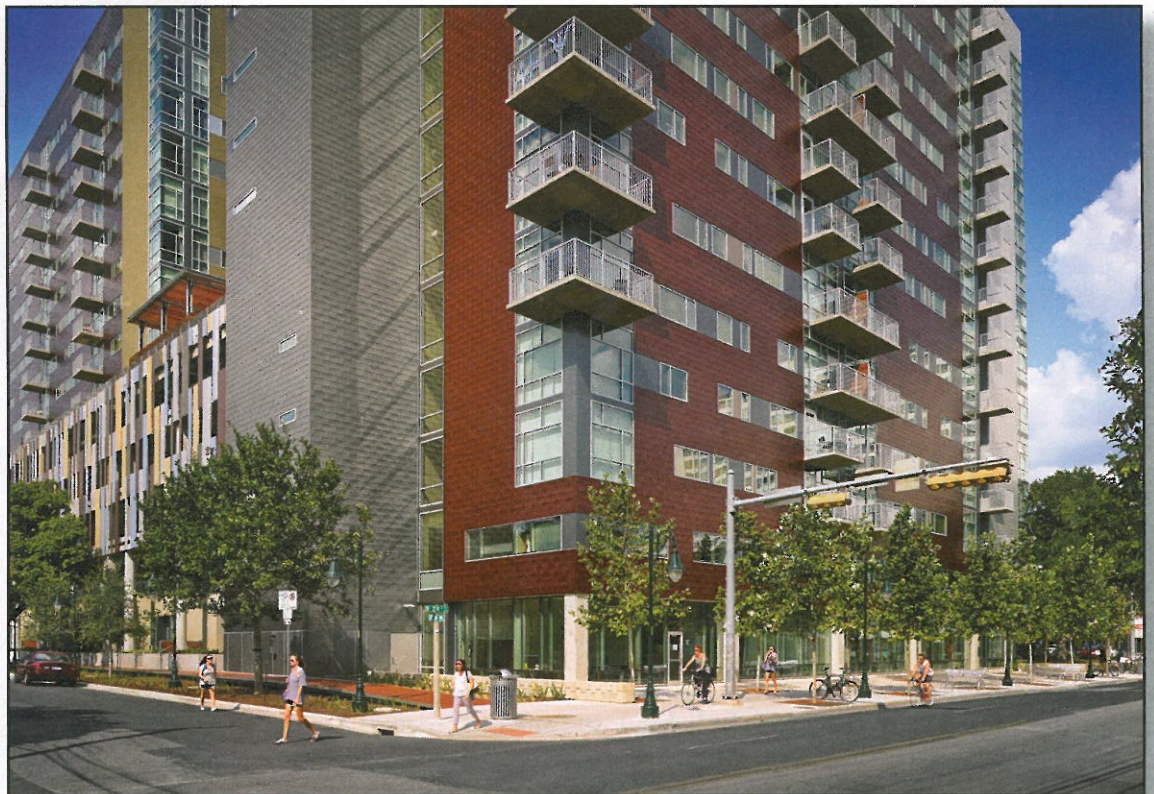
EdR developed, financed, owns and manages 2400 Nueces, a 304-unit, 622-bed, 16-story community.
